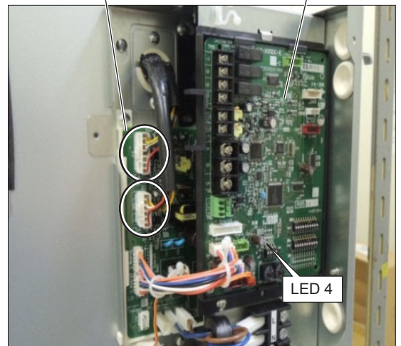
Power circuit board Control circuit board
