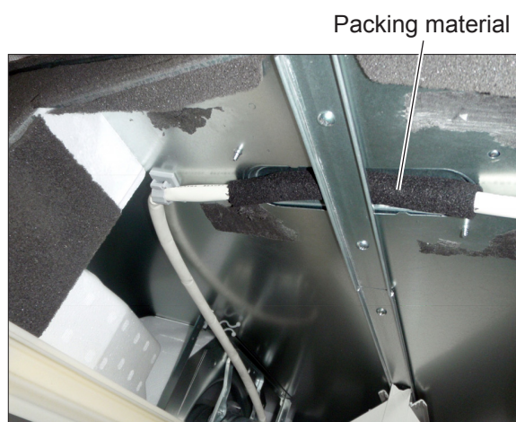
<After replacing the motor>
