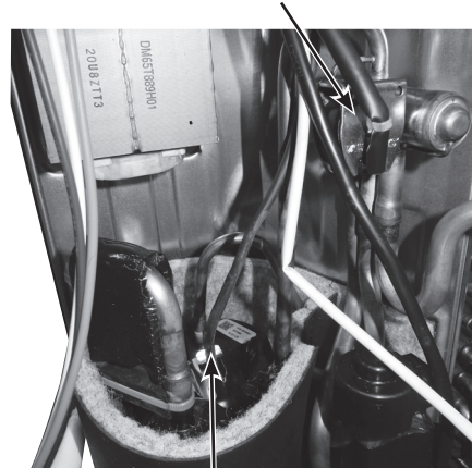
Discharge temperature thermistor
